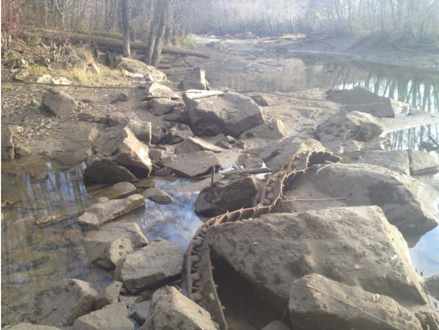
Photograph 13: Metal Debris at Stream.
