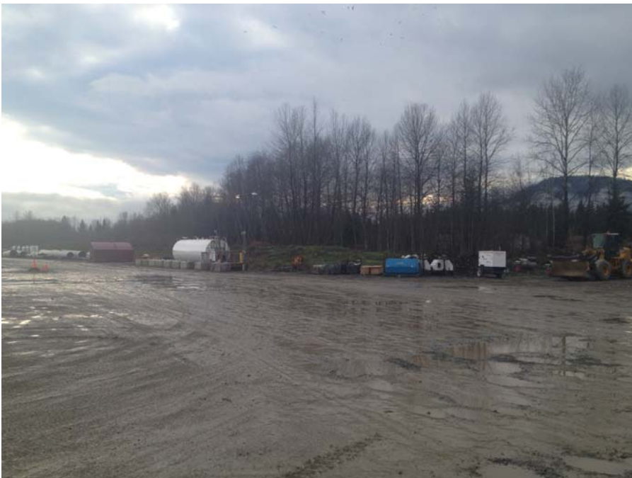
Photograph 18: Valard Laydown Area with AST.
