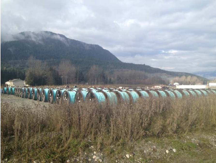
Photograph 17: Valard Laydown Area.
