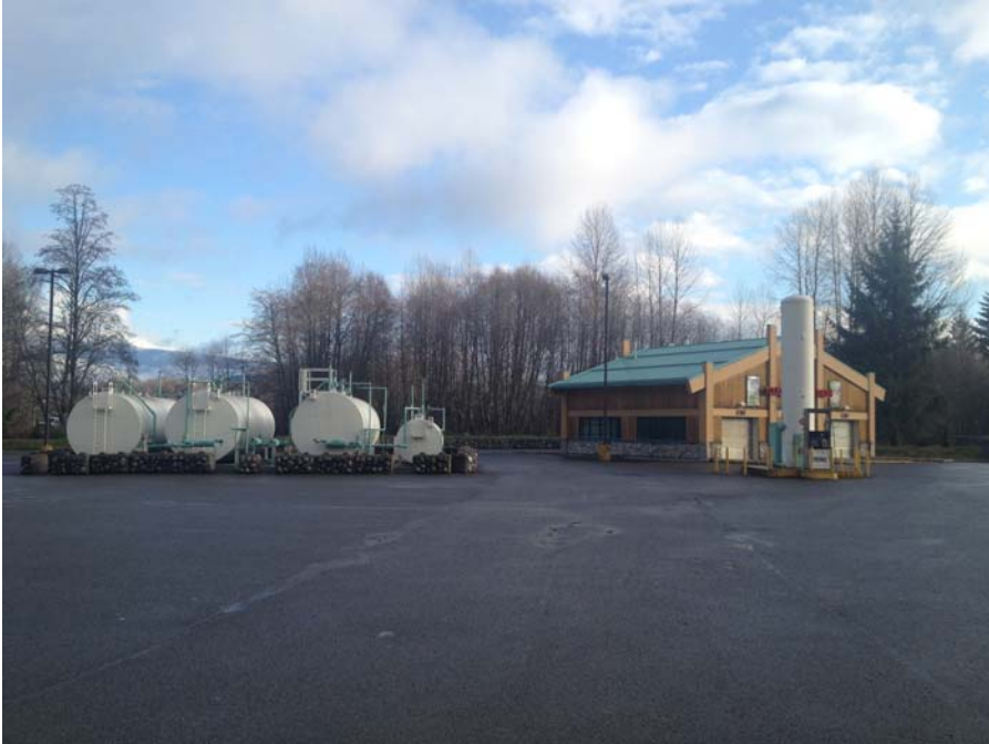
Photograph 23: Tempo Gas Bar ASTs.
