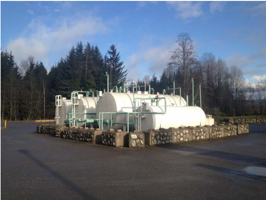
Photograph 24: Tempo Gas Bar ASTs.
