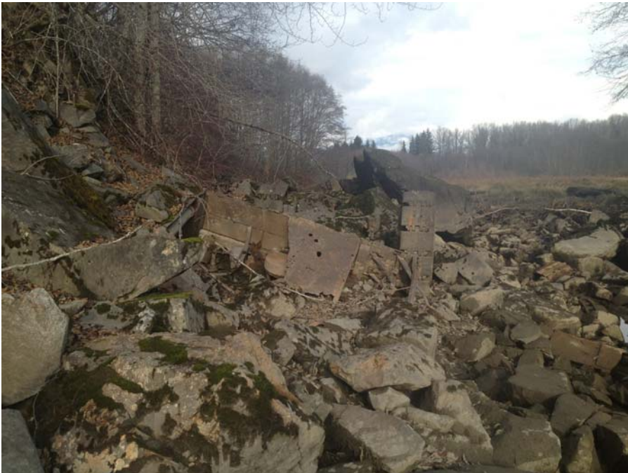
Photograph 14: Metal Debris at Stream.
