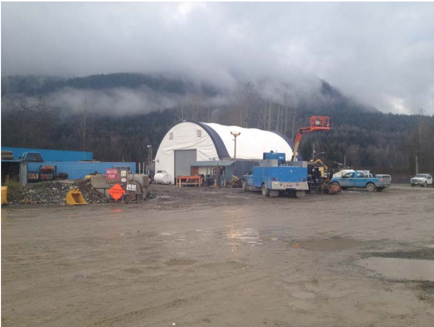
Photograph 16: Valard Laydown Area.
