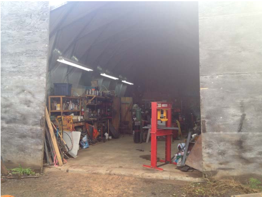
Photograph 2: Band Maintenance Shed Entrance.
